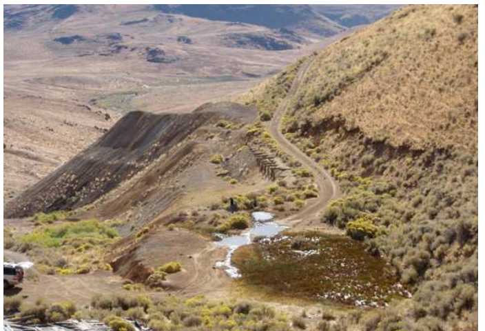
The mine entrance has long been walled up. The hillside is sliding down and polluted water drains out. Below is a view of the mine area. The swamp area is from the mine drainage. In the center to the left of the roadway is the remains of the ore car trestle.
