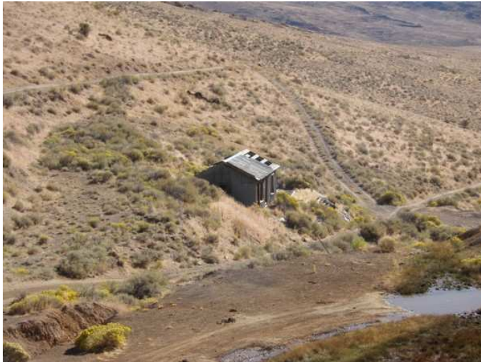
The mine entrance has long been walled up. The hillside is sliding down and polluted water drains out. Below is a view of the mine area. The swamp area is from the mine drainage. In the center to the left of the roadway is the remains of the ore car trestle.
